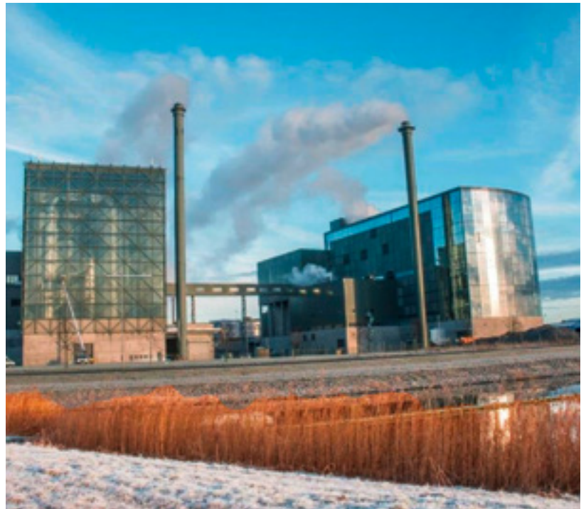
The trash-powered plant in Linköping, in Sweden, which generates electricity and heats water for home and commercial use, harnesses 90 percent of total energy. This centralized system of "district heating" warms many buildings in Sweden.
